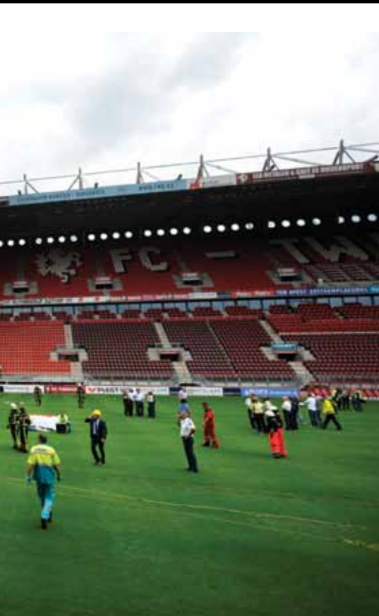
Figure 1 Collapse resulted in two fatalities and nine injuries
