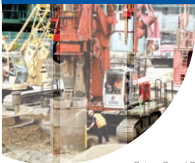
Rotary Bored Piles in Wimbledon
