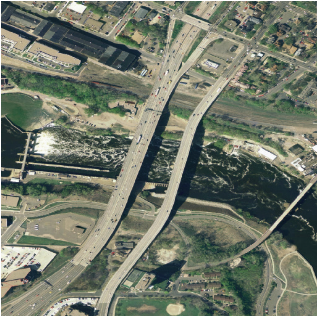
Aerial view of the I-35W Mississippi River Bridge and the surrounding area. The bridge collapsed in August 2007. Just to its right is the older 10th Avenue Bridge. Credit: U.S. Geological Survey
