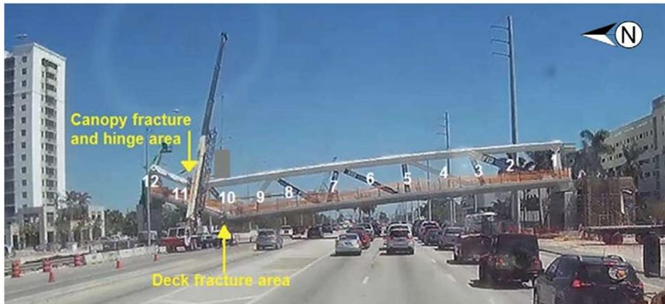
Figure 5 Fracturing of bridge (NTSB, 2019)
