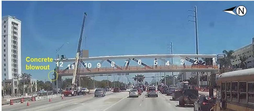
Figure 4 First sign of failure (NTSB, 2019)
