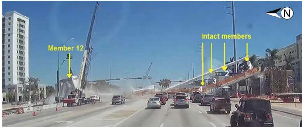
Figure 6 Final collapse (NTSB, 2019)
